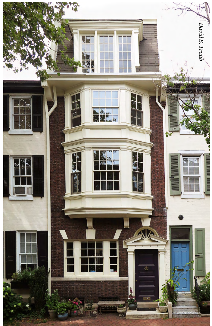
House on 2200 Block of Rittenhouse Street (p. 16)
